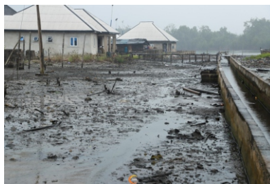
► Waterlogged ground stretches between homes and a creek in Bille, where gas has been bubbling through the soil and nearby water bodies
