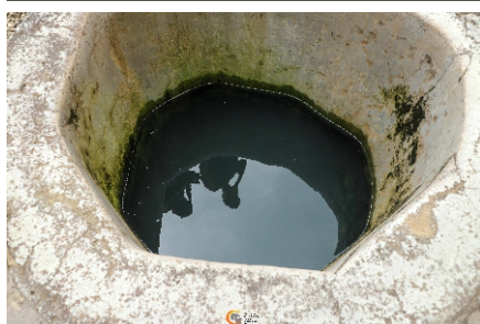
Dark, contaminated water inside a well in Bille.
